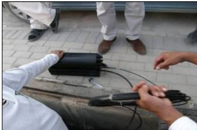
Pre-connectorized Network Access Terminals deployed like standard closures
