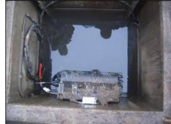
Pre-connectorized Network Access Terminals deployed like standard closures
