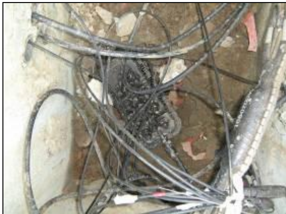
Pre-connectorized Network Access Terminals deployed like standard closures
