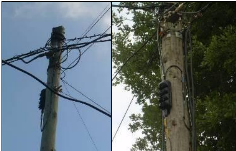
Multiport with loop of tether & stub cable
