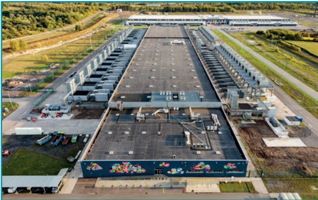
Google data centre, St. Ghislain, Belgium [credit: Google]
