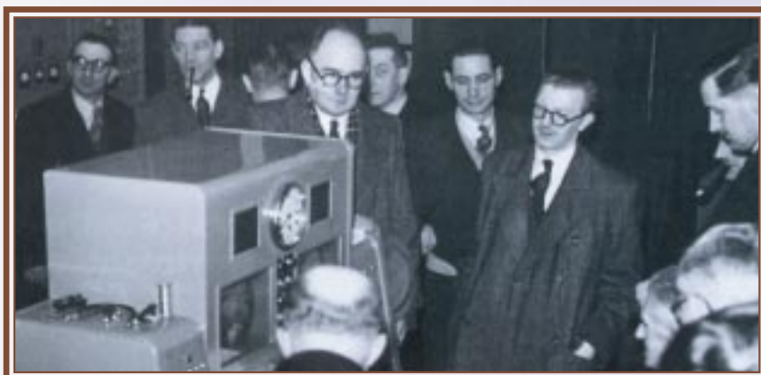
February 26th 1952: SRE members visiting the relay station of Britain's first cable TV system at Gloucester, then owned by Link Sound & Vision Services Ltd and later acquired by British Relay Wireless Ltd. Signals from Sutton Coldfield at Chosen Hill were beamed by a parabolic VHF antenna to an amplifying station in the city and then to subscribers on a 10MHz carrier. Subscribers could have either four sound programmes or three sound programmes and television.
